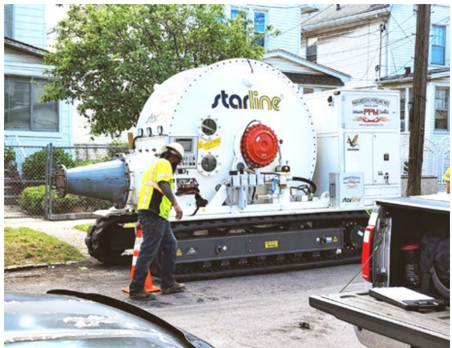
The Starline® Cured-in-Place-Lining Inversion Drum on 134th Street
