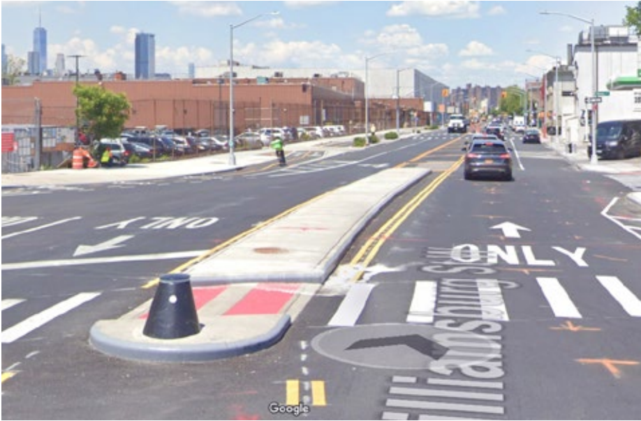
Concrete Median in Williamsburg, Brooklyn and site of the Chair Challenge
