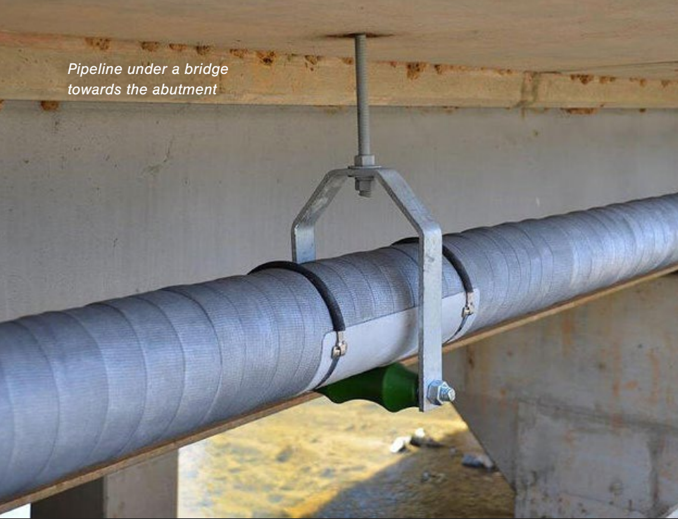
PPM Crew installing SRS sleeve between abutment wall and gas main
