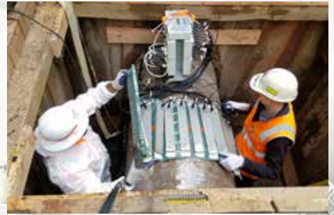
The Flexible Array Scanning Tool (FAST) external ferrous wall condition assessment.
