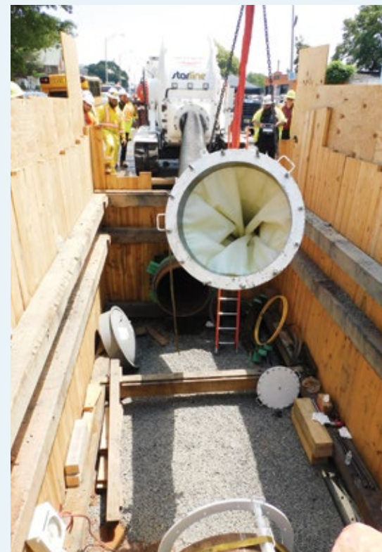
Leaking 42-inch cast iron gas main repaired using Starline® Cured-In-Place-Lining (CIPL)
