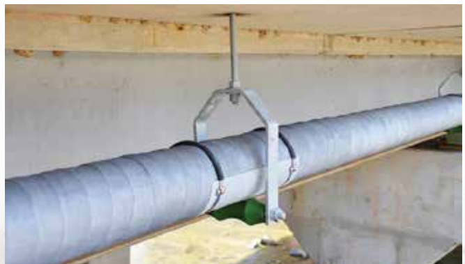
Figure C. Pipeline under bridge going towards abutment
