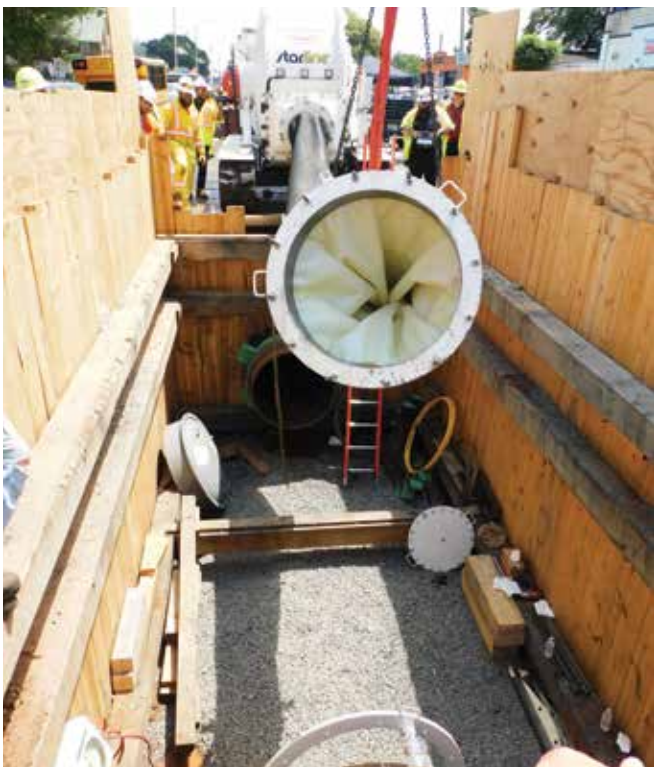
Figure J. PPM Cured-in-place-liner inversion in process
