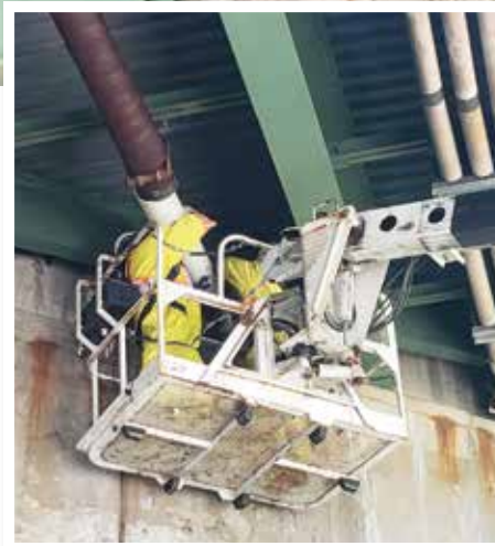
Figure G. PPM crew installing SRS sleeve and PVC pipe between abutment wall and gas main
