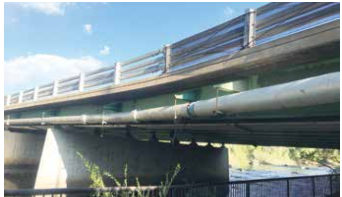
Figure B. Bridge with pipeline alongside
