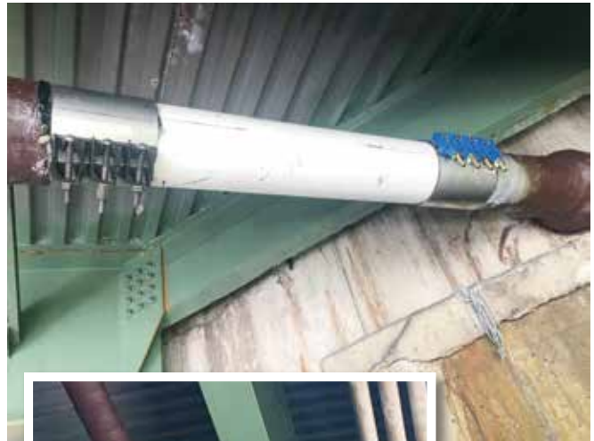
Figure G. PPM crew installing SRS sleeve and PVC pipe between abutment wall and gas main
