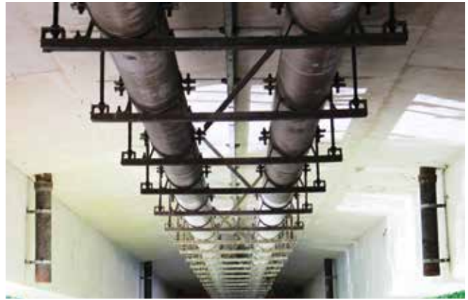
Figure A. Bridge with pipeline hanging under bridge
