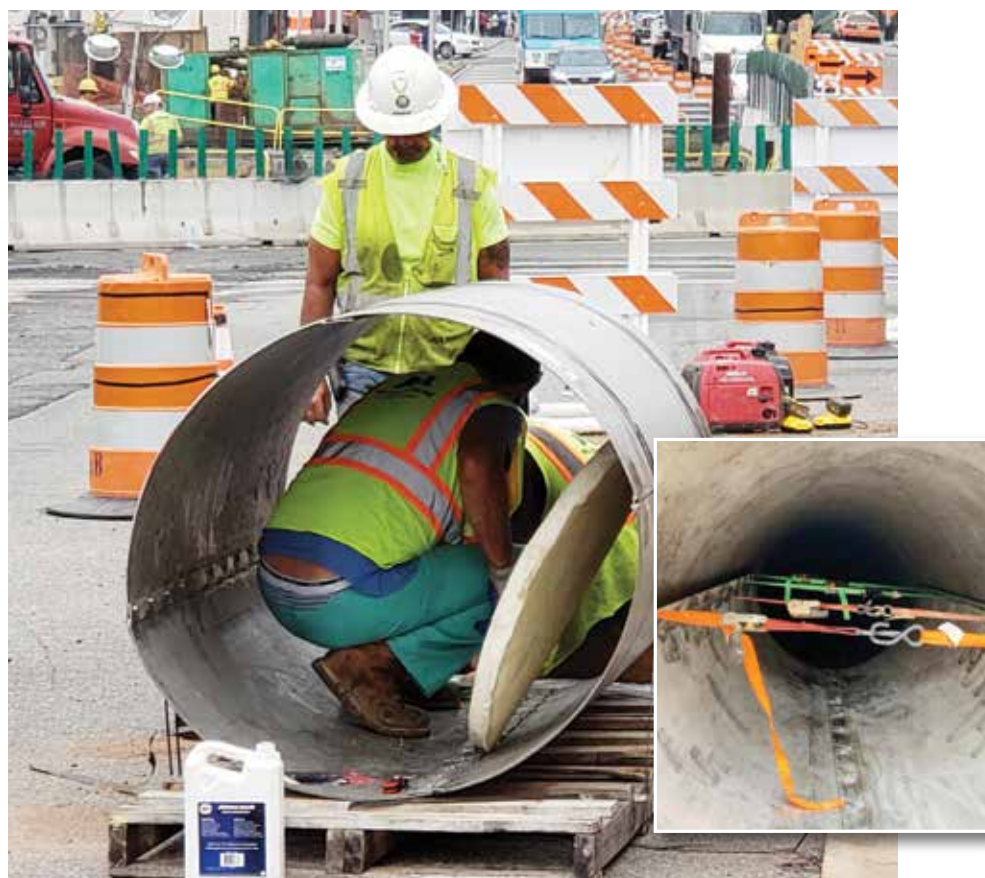
Resourceful Miller Pipeline crew successfully installed largest SRS bridge ever fabricated
