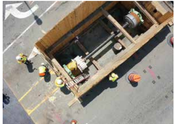
Receiving pit, Central Avenue West
