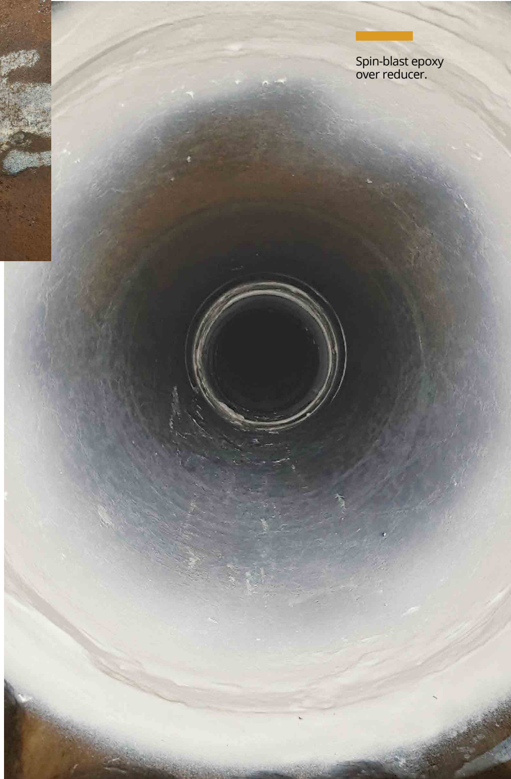
30 in (760 mm) diameter gate valve well.
