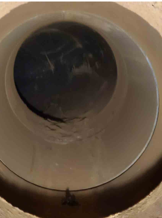
30 in (760 mm) diameter gate valve well.
