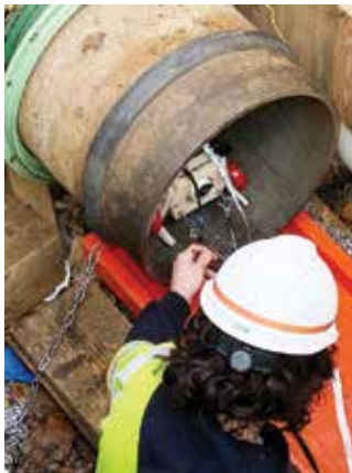
Figure 2. BEM internal tool inserted into 20-inch cast iron main
